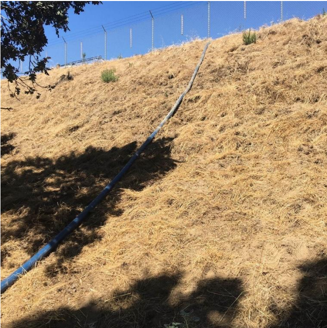
Photograph 3 - August 2, 2019 Seepage Water Pumping Back into Basin 4, Photo Shows High Elevation Difference from Treatment Facility to Offsite Property, which Accelerates Seepage
