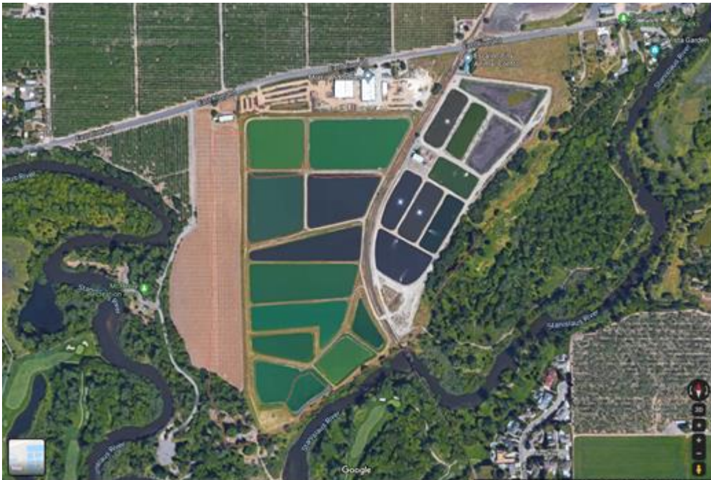
Figure 1 – Aerial Google Image of the Escalon WWTP: +/-28-acres of Treatment Basins 1-9 (right), +/-15-acres of Domestic Percolation Basins (four large square basins in upper left), and +/-23-acres of Industrial Percolation Basins (remaining 8 basins in lower left)
