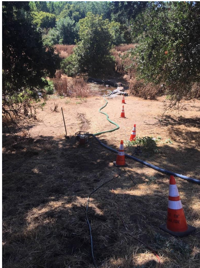
Photograph 2 - August 2, 2019 Side Wall Seepage of Industrial Treatment Basin 4 to Offsite Property Due to Unlined Earthen Basins Situated High Above Adjacent Property
